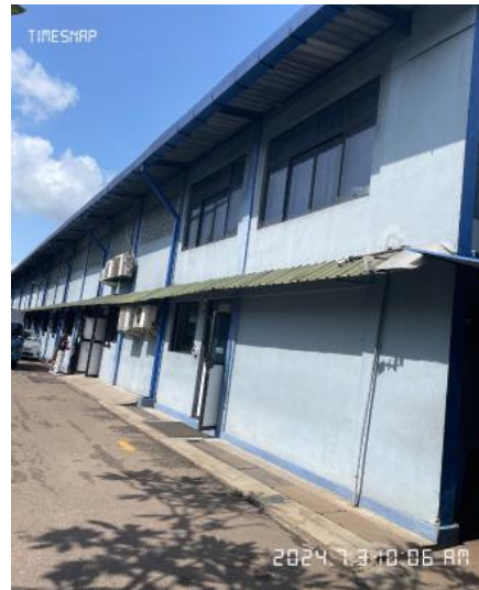
4.Side view of the facility.JPG
