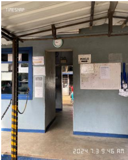
3.Security post near entrance.JPG
